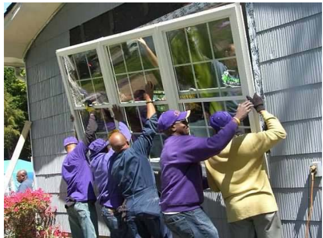
Mu Rho Brothers replacing a window. Working Hard for Omega
